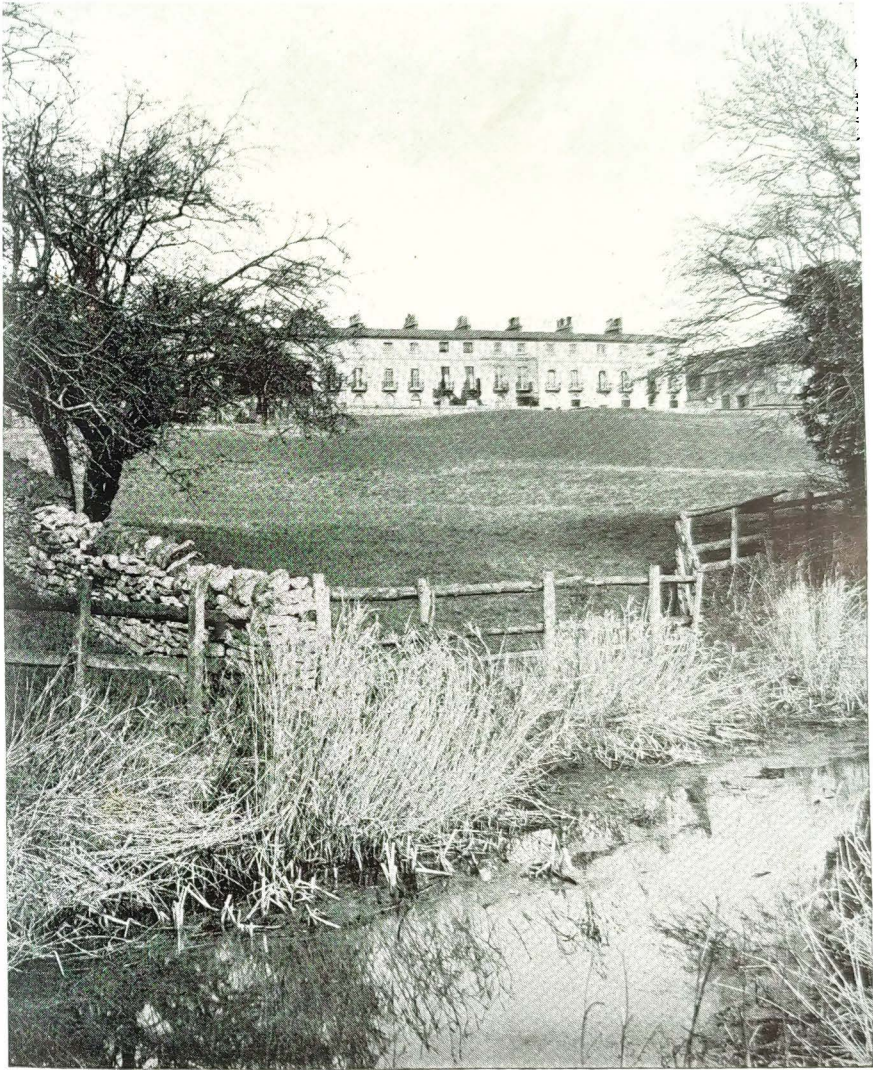
RUTLAND TERRACE, as seen from Melancholy Walk, across the site of Austin Friary.
