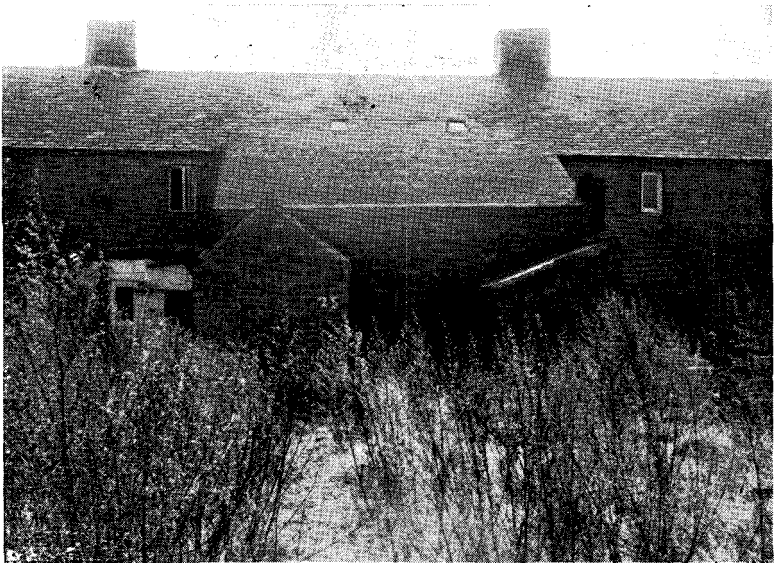
REAR OF NO. 25, PORTLAND ROW. The Chapel, of which only a part remained when this photograph was taken, originally extended a further 20 feet over the ground in the front of the picture.
