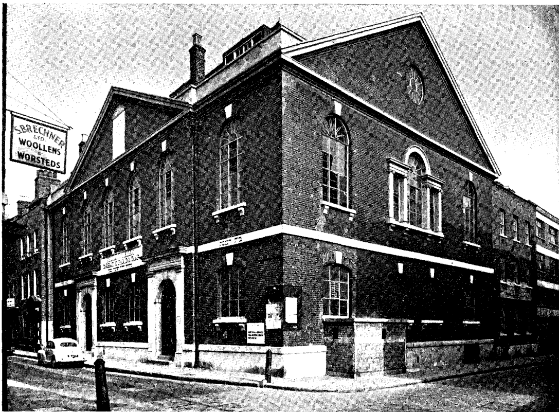
THE FORMER WESLEYAN CHAPEL IN FOURNIER STREET (THEN CHURCH STREET), LONDON (now a Jewish Synagogue).
