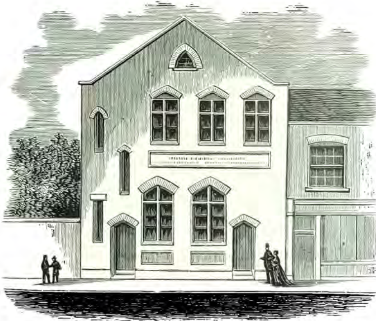
THE OLD BUILDING.
