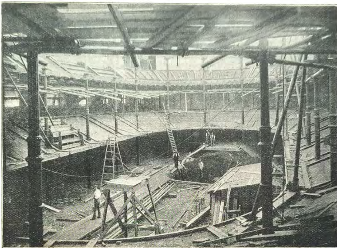
THE METROPOLITAN TABERNACLE,—PROGRESS OF REBUILDING AFTER THE FIRE.
