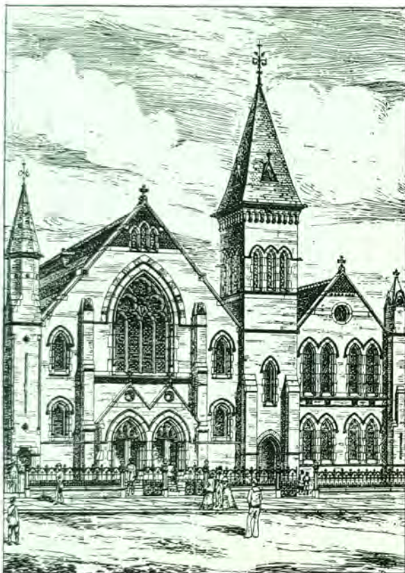
CEYLON PLACE BAPTIST CHAPEL, EASTBOURNE.
