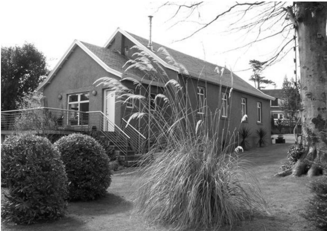
A view from the rear of the second Kames Free Presbyterian building, now converted into a dwelling house.
