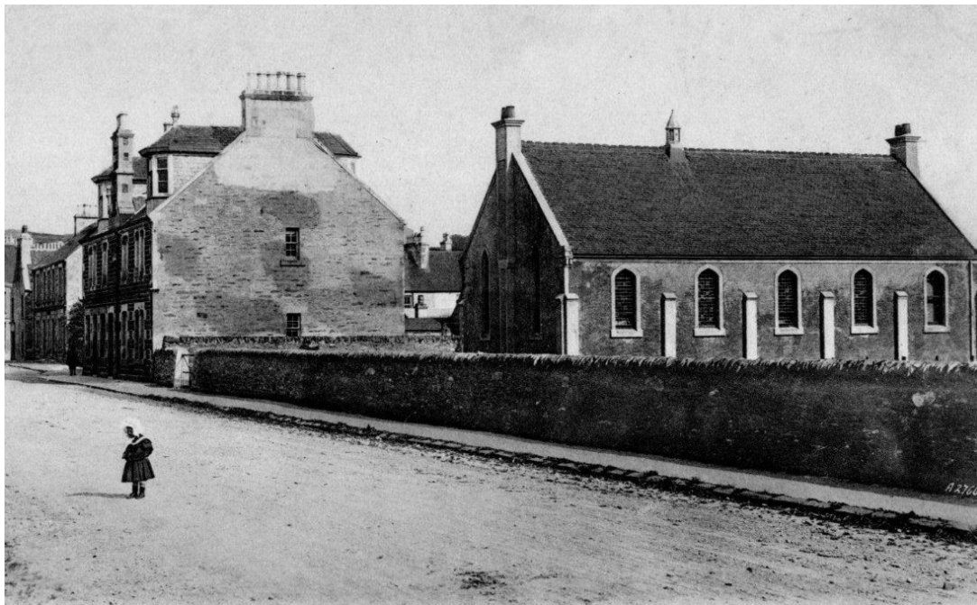
The Lochgilphead Free Presbyterian Church building stood on Lorne St. in the town and was paid for by members of the congregation and friends across mid-Argyll and further afield. It was shut down in 1973 and demolished soon afterwards. A telephone exchange was built on the site.
