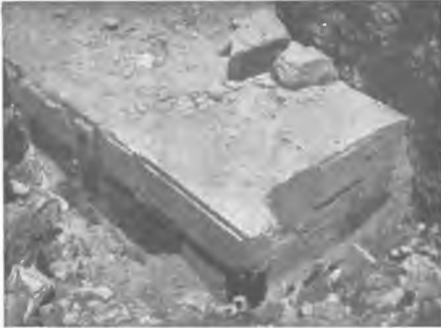
10. WESTERN PIER, FROM THE SOUTHWEST.
