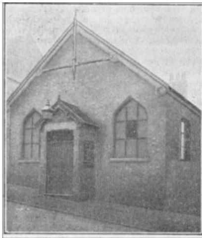
Elim Hall, Ashbourne
