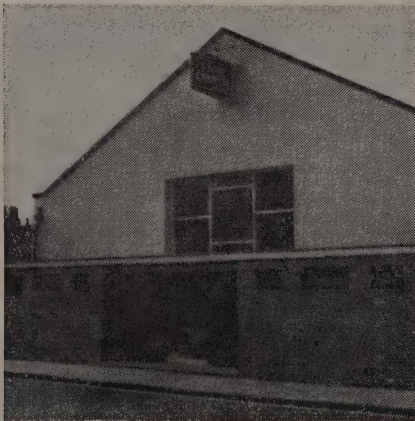
The new front of the Portsmouth church.
