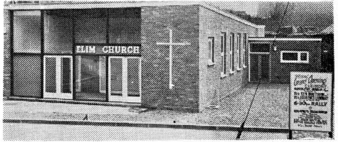
Front view of church.
