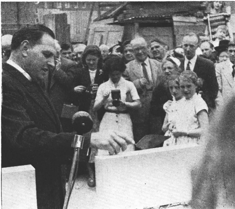
Pastor F. Hodge laying one of the Foundation Stones.
